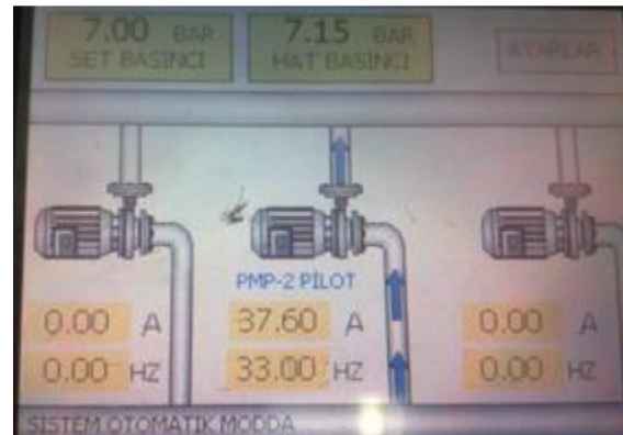
Figure 5. PLC used in an irrigation pumping plant
